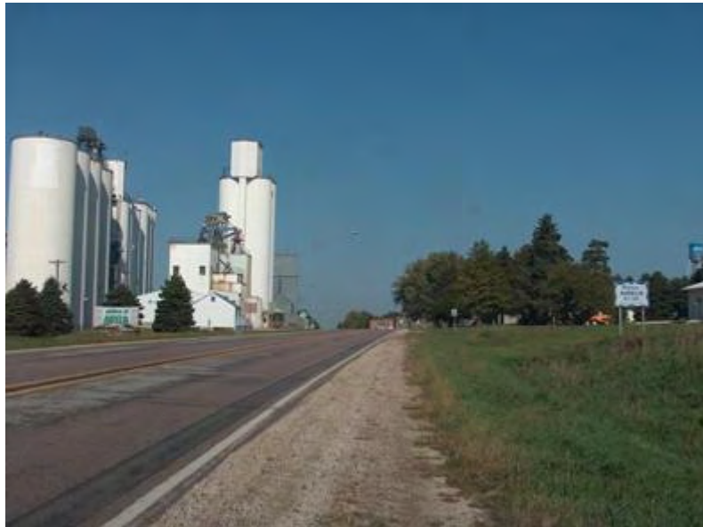
Figure 1.1. Major highway entering a small Iowa community
