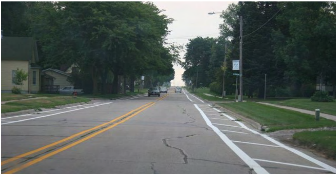
Figure 3.34. Use of shoulder widening in Roland, Iowa as part of gateway treatment
