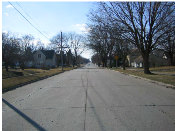
Figure 5.18. East side of E-18 before lane narrowing
