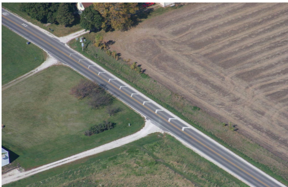
Figure 5.21. Aerial view of Roland treatment
