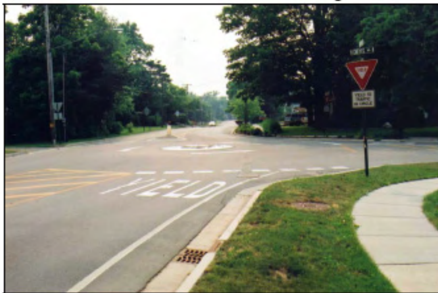
Figure 3.44. Another view of the Dimondale, Michigan installation
