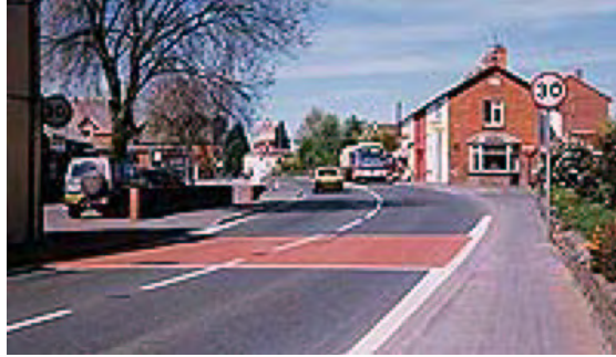
Figure 3.29. Treatment used in Shropshire, UK (source: DETR 2005)
