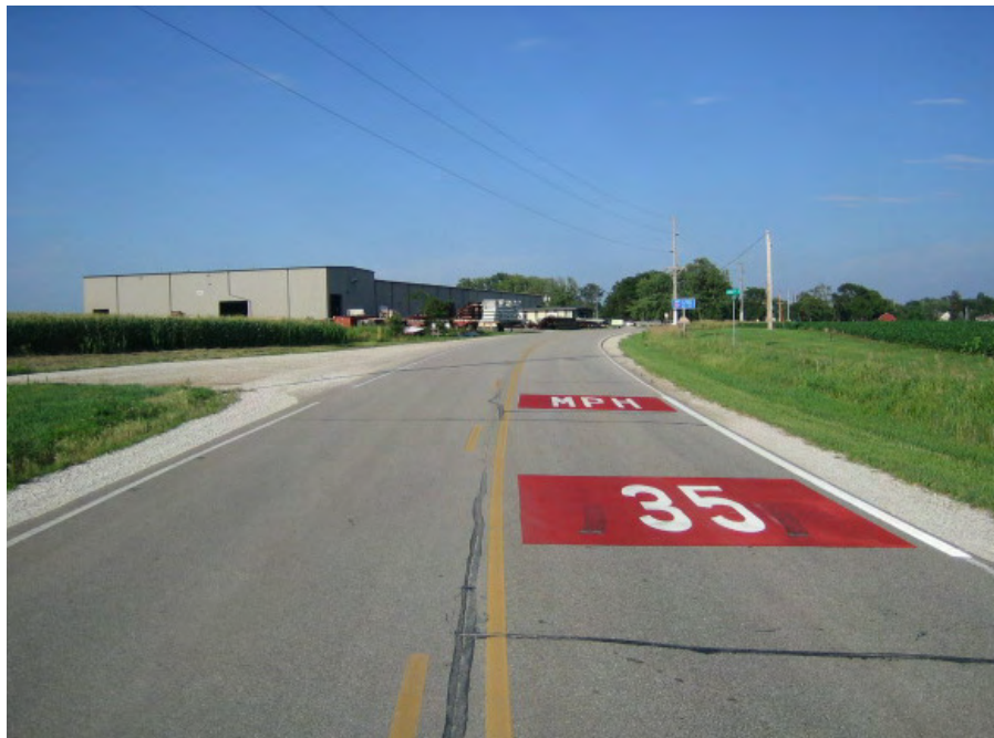
Figure 5.42. After installation of treatment before industrial plant
