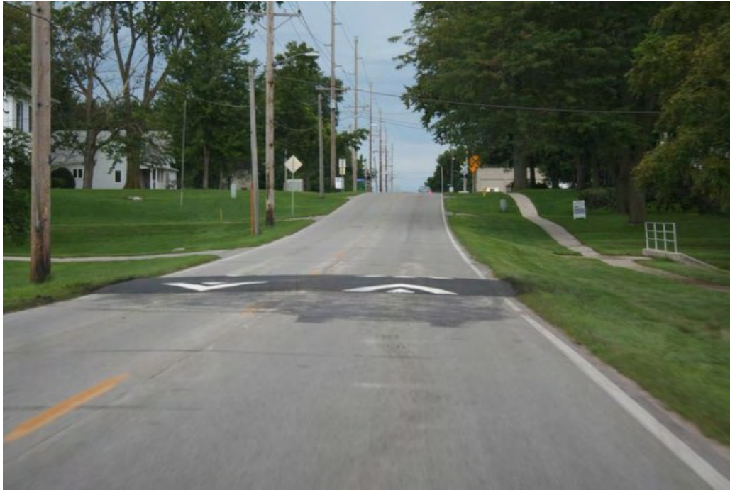
Figure 5.27. Gilbert after installation of speed table
