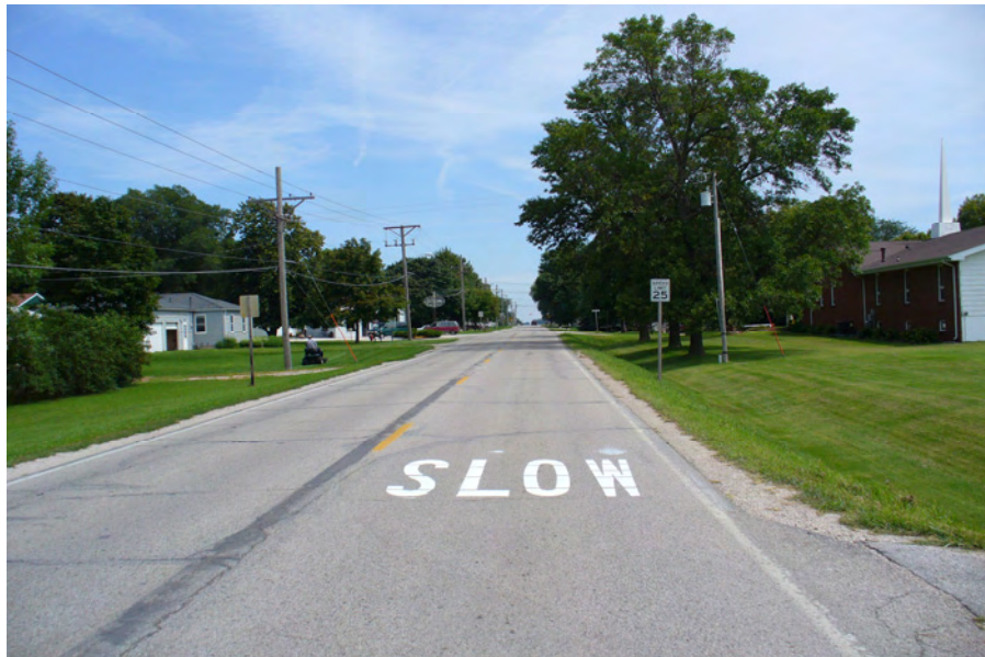
Figure 3.38. Use of on-pavement “SLOW” marking around a pedestrian crossing area in Slater, Iowa
