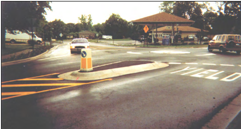
Figure 3.42. Mini-roundabout in Michigan
