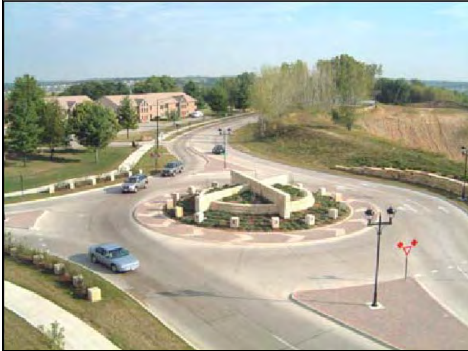
Figure 3.39. Roundabout in Coralville, Iowa (source: Runge 2005)
