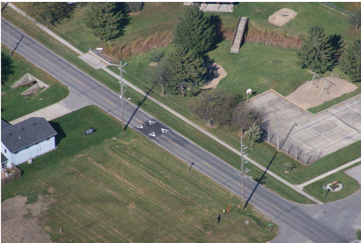
Figure 5.28. Aerial view of speed table
