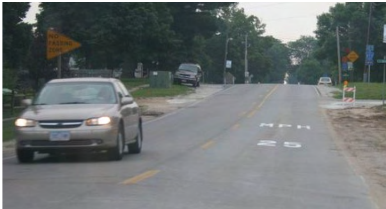
Figure 3.37. Use of on-pavement speed markings in Roland, Iowa as part of a gateway treatment
