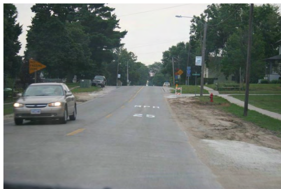
Figure 5.20. On-pavement speed signing
