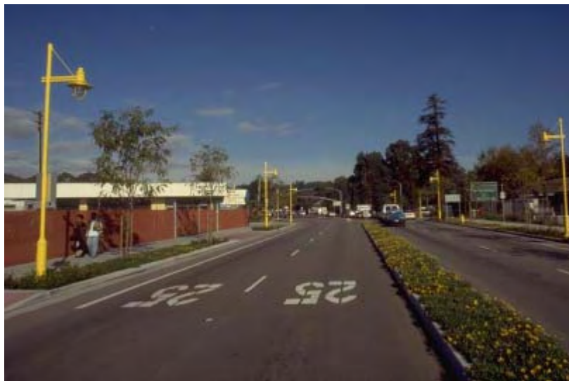
Figure 3.36. Speed limit pavement markings (source: CWS 2005)
