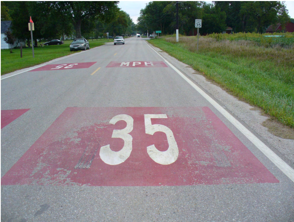
Figure 5.45. Wear of Dexter treatment over time.
